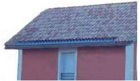
Fitting at the gutter
